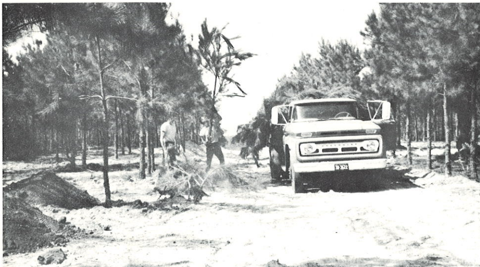
Work nears completion in the Pine Orchard. Campers will be pleasantly surprised when they see the wonderful facilities that have been constructed!
